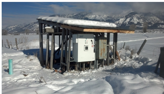
Variable frequency drive and transducer installed as part of the Agricultural Efficiency Program
