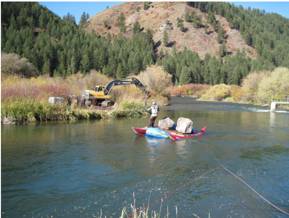
Fish ladder construction at the East Side Canal, Salt River.
